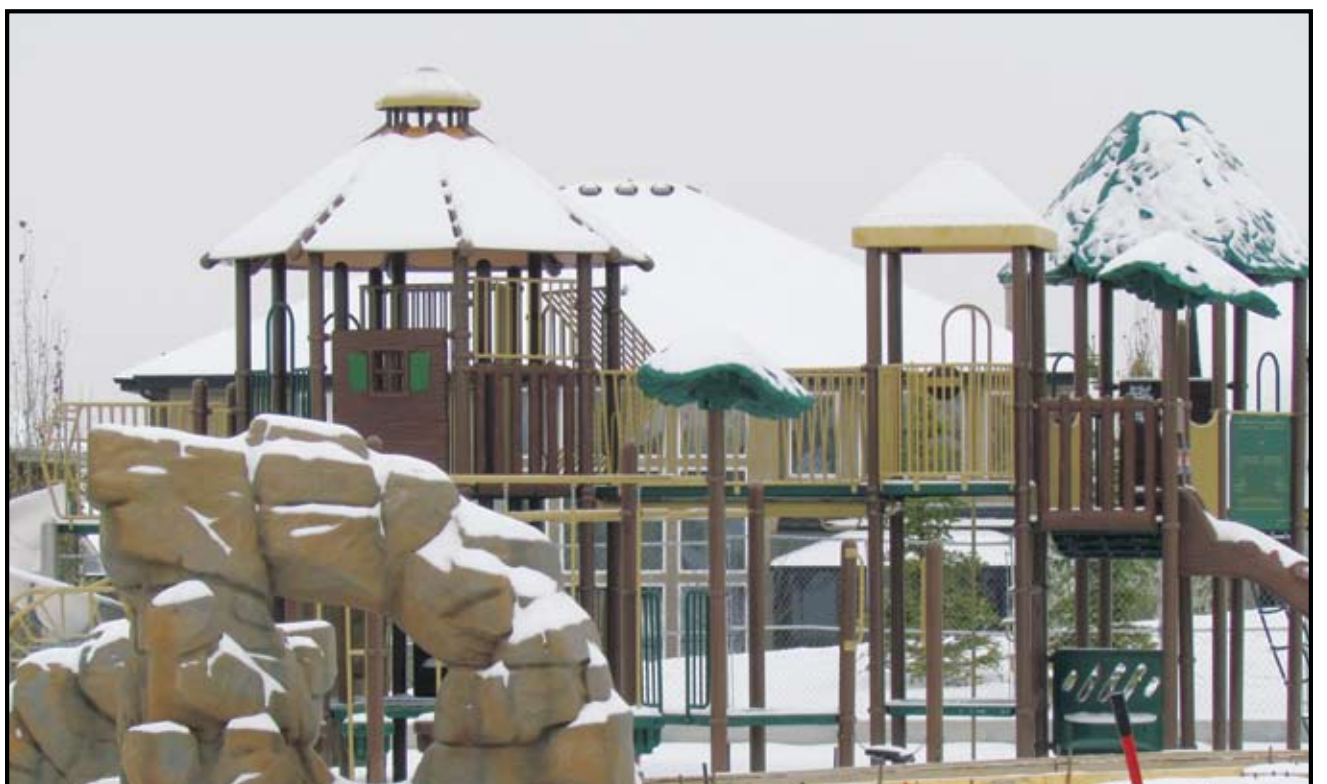
Magrath park site is currently under construction. Thank you to the volunteers, sponsors and donors who made this playground possible. Photo by Danielle Gordon.
