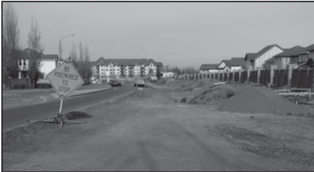
Widening of Rabbit Hill Rd. continues.
