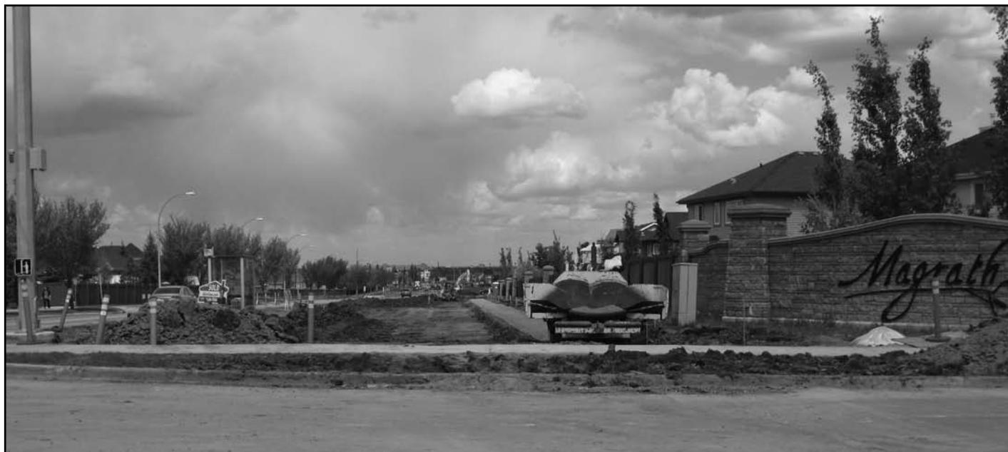
Looking north toward 23 Ave. from Magrath Blvd. — Rabbit Hill Rd. construction continues this summer.
