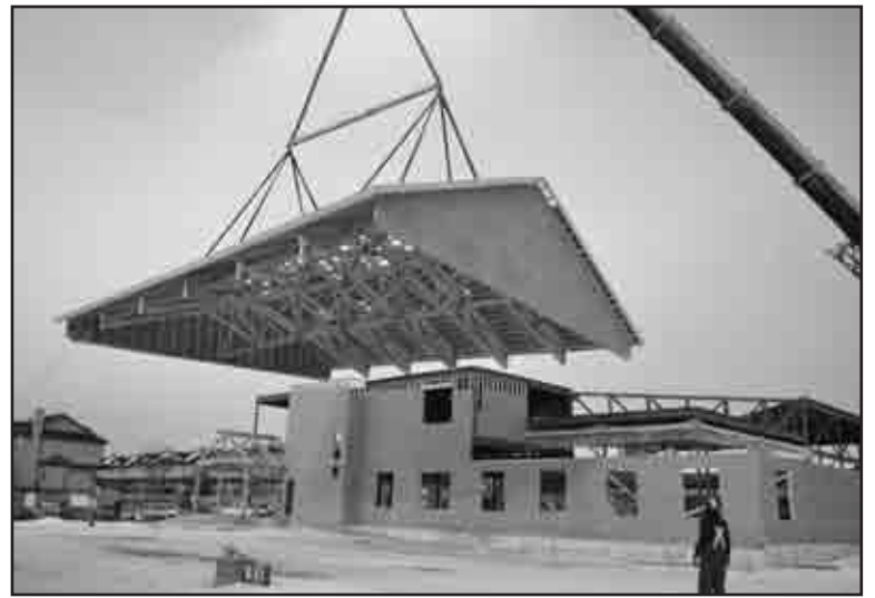
The new Terwillegar Community Church may open as early as May.
