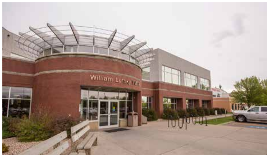
SWESA's new home within the Y. Photo credit: Hendricks Construction
