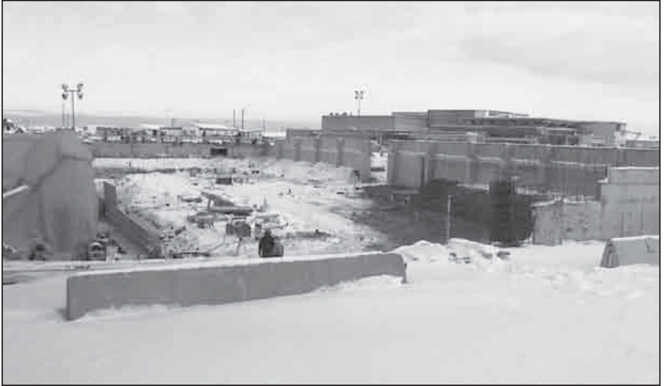
Above: The SCRC begins to take shape as the foundation walls for the pool basin are formed.
