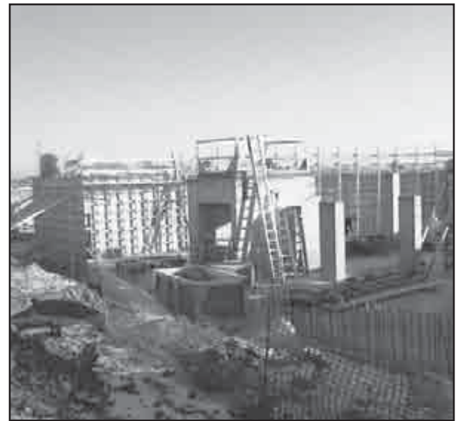
Above: Construction takes place on the lower mechanical room elevator shaft.
