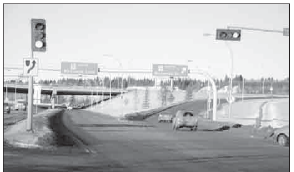
This ramp, from Fox Dr. onto Whitemud Dr. westbound (here indicated north), will be closed to traffic from March until October or November.
