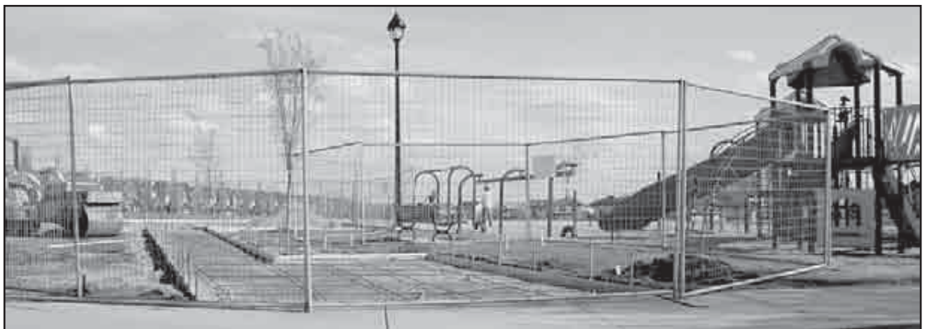
Fences surround the construction area for the safety of all visiting the park.
