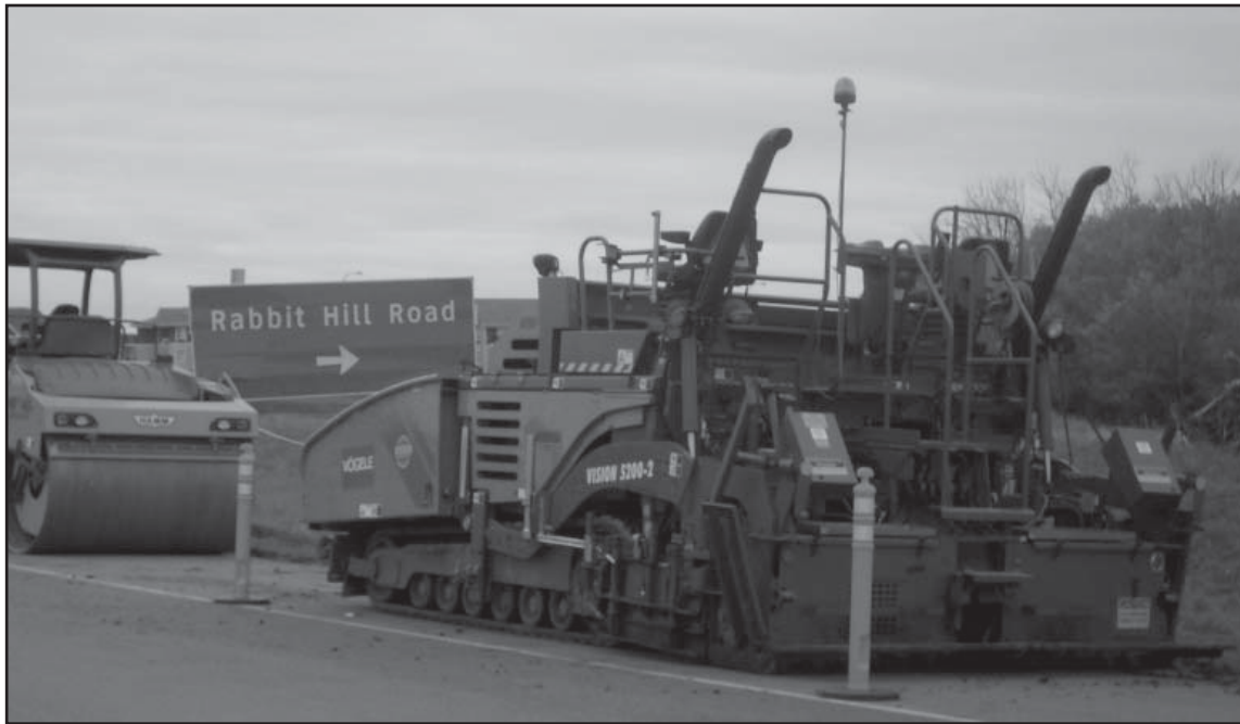
On May 26, it was announced that construction is underway on the Rabbit Hill Rd. overpass at Anthony Henday Dr. The project is to be completed in fall 2011.
