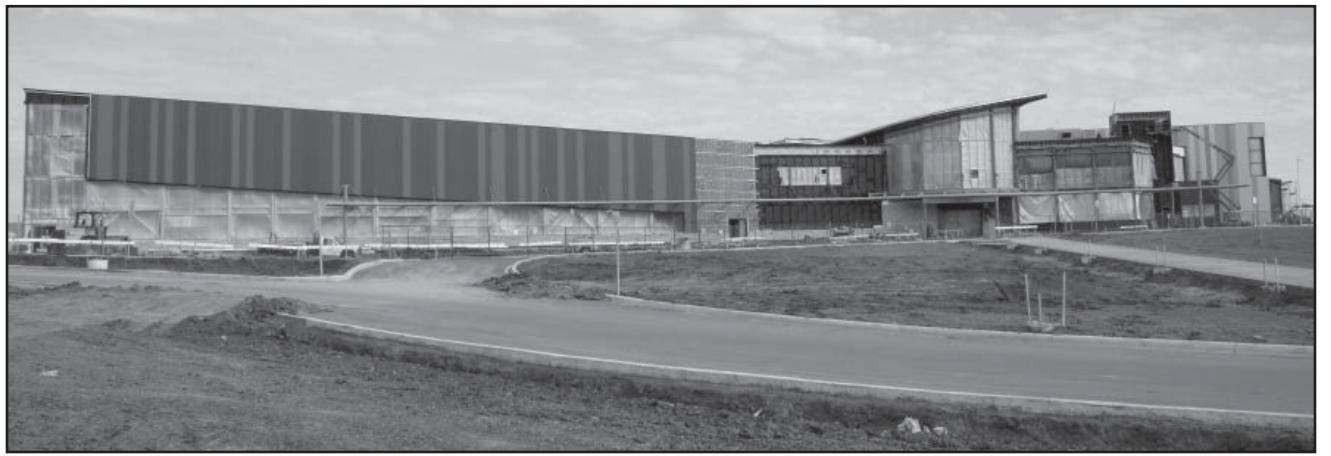
Red and beige aluminum cladding starts to bring the recreation centre to life.
