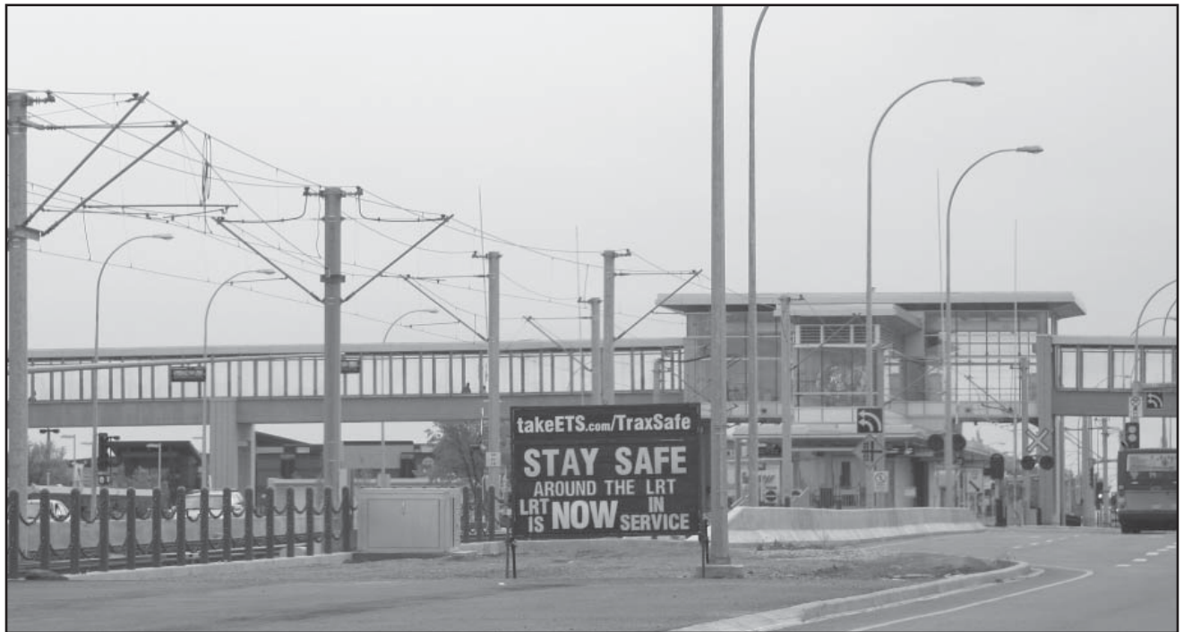
The City of Edmonton warns pedestrians to stay safe around the newly constructed Century Park LRT station.
