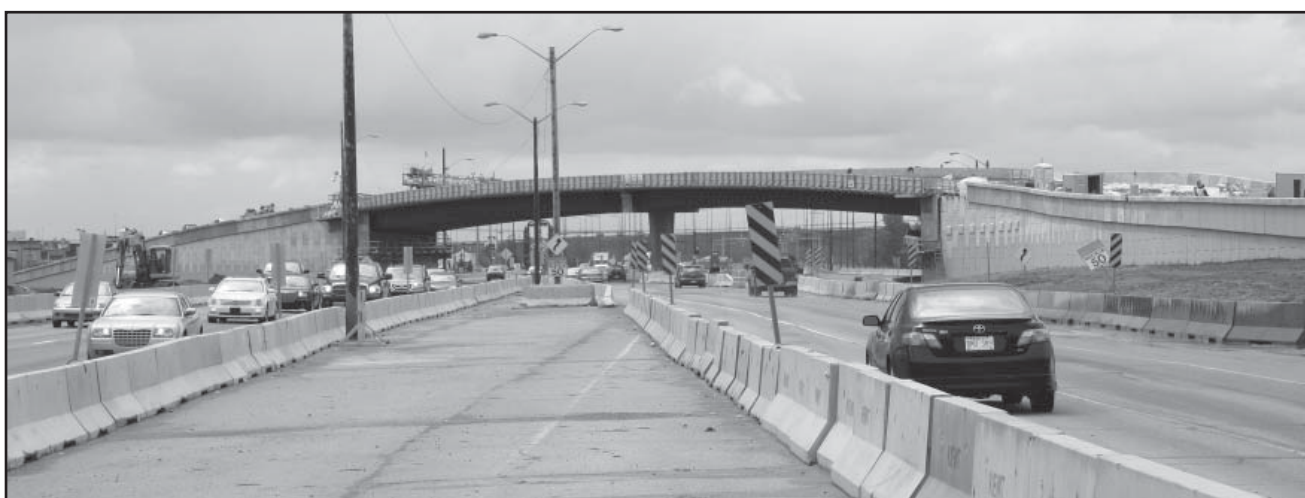
Construction continues on the 23 Ave./Calgary Tr. Interchange.
