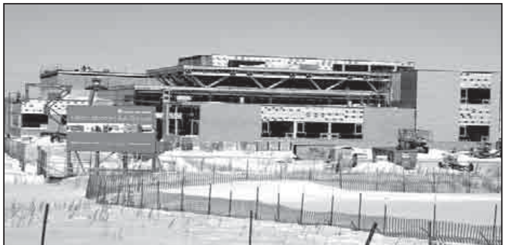
The Lillian Osbourne High School is set to be completed by September 2009.
