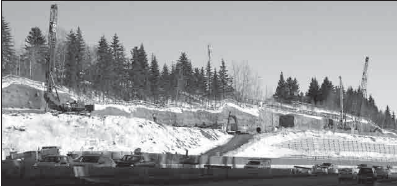
Above: Work progresses on the Quesnell Bridge widening.
