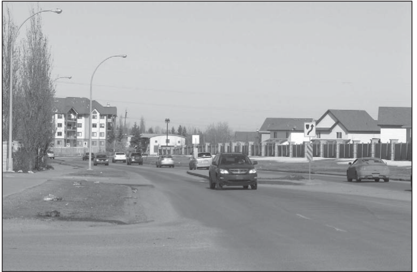
Construction on this area, Rabbit Hill Rd. north of 23 Ave., is expected to start in 2011. The road will should be widened to four lanes.
